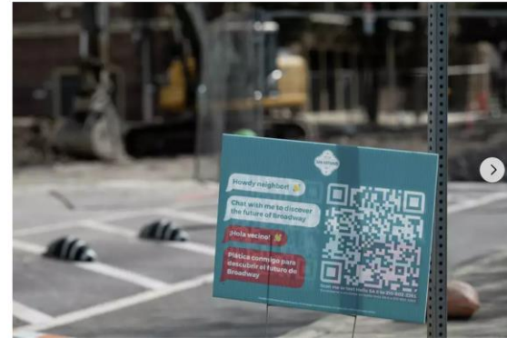
A sign with QR codes telling people about a chatbot that responds to questions about construction along Broadway at the corner of McCullough Ave and Broadway on Saturday, Jan. 13, 2024 in San Antonio. There are 40 signs all along lower Broadway Salgu Wissmath/San Antonio Express-News
